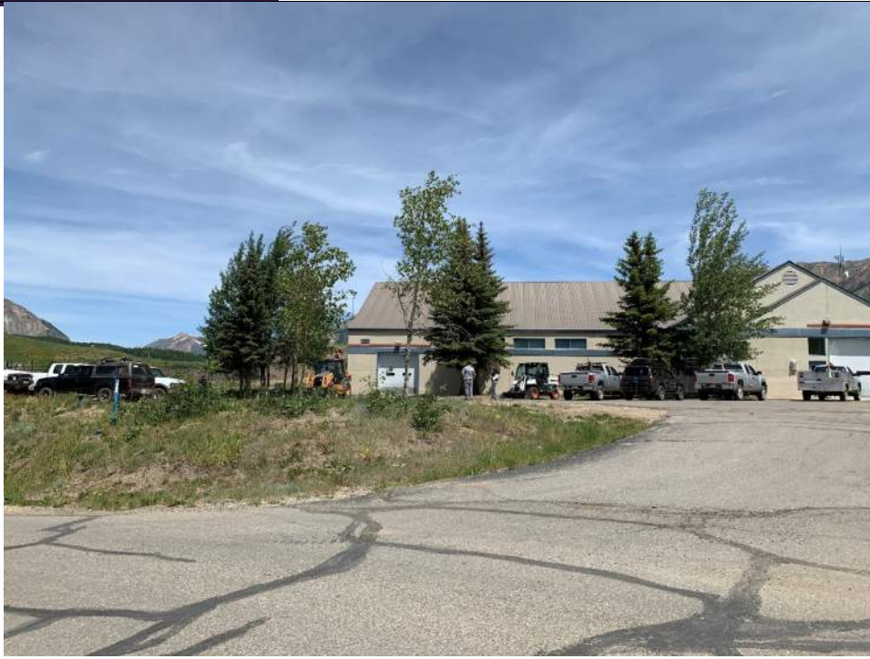
3. Existing Water Treatment Plant (Facing North)
