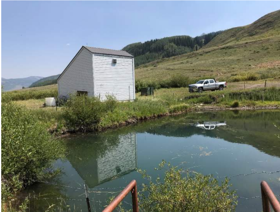
1. Existing Pump Station and Pre-sedimentation Pond (Facing Northeast)
