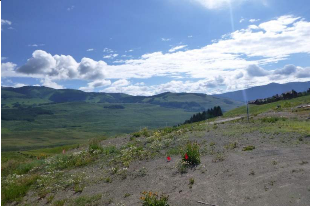
Figure 2. Project overview, view to the east. Photo number: P1040060.jpg Date: 8/8/2019
